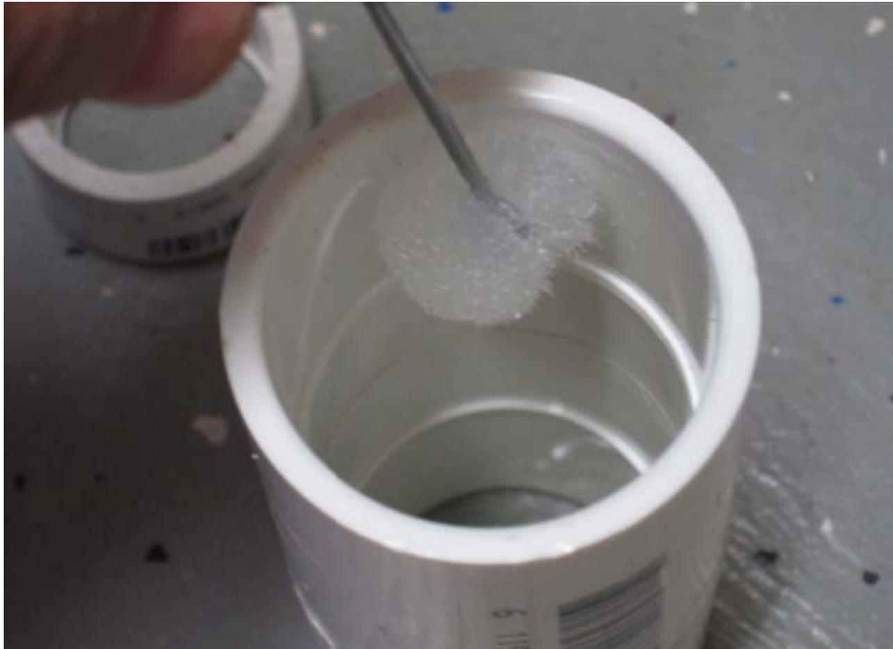
Invert the coupling and press the glued end down carefully over the bushing.
